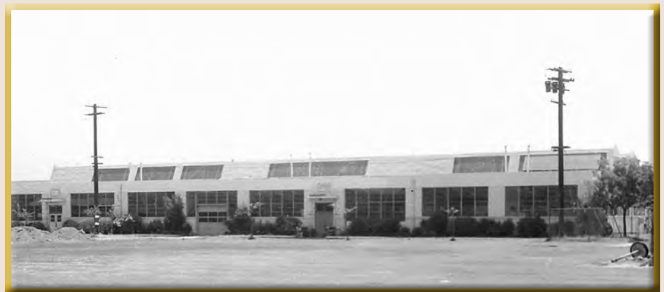
Printing, Painting, Carpentry and Wood Working
